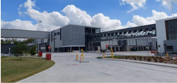
Heathwood Chilled & Frozen DC, Qld New manual chiller and freezer facility Opened ahead of schedule in H1
